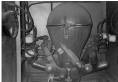
Mercury Arc Valve
