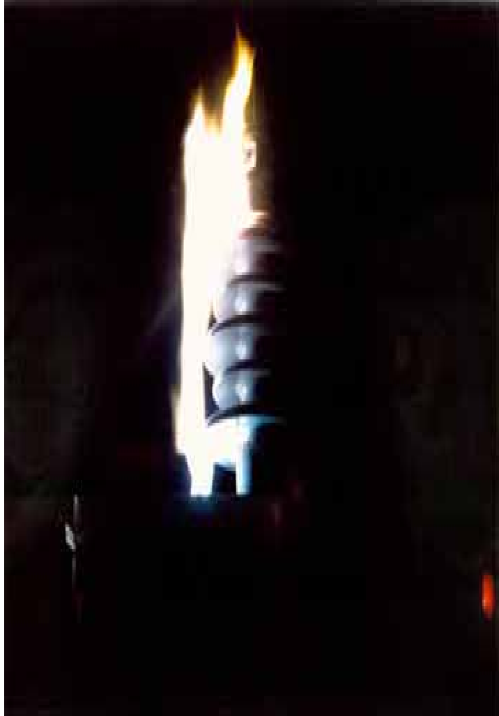
Figure 1.2: The picture of a flashover of an insulator [5].
