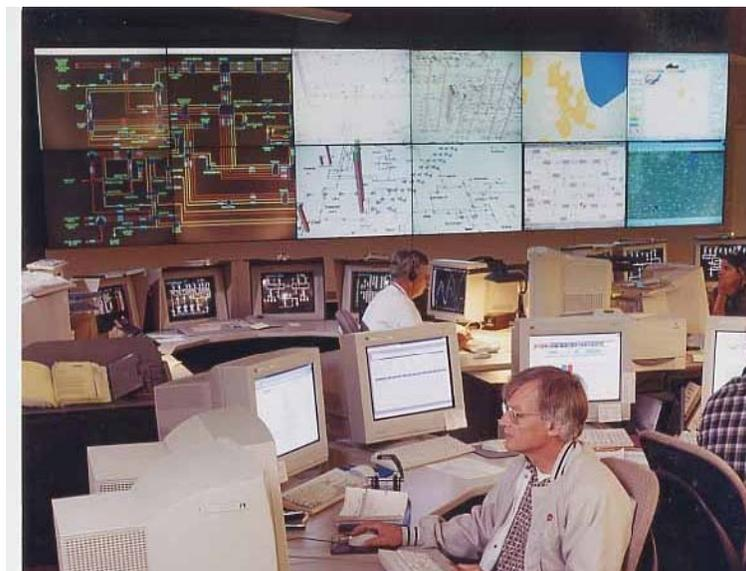
*Figure 6: Commonwealth Edison Control Center in Northern Illinois.* Control centers are busy places, with data coming from hundreds of sources that has to be quickly processed and interpreted. Visualization tools contribute to turning data into “information” useful for decision-making.
